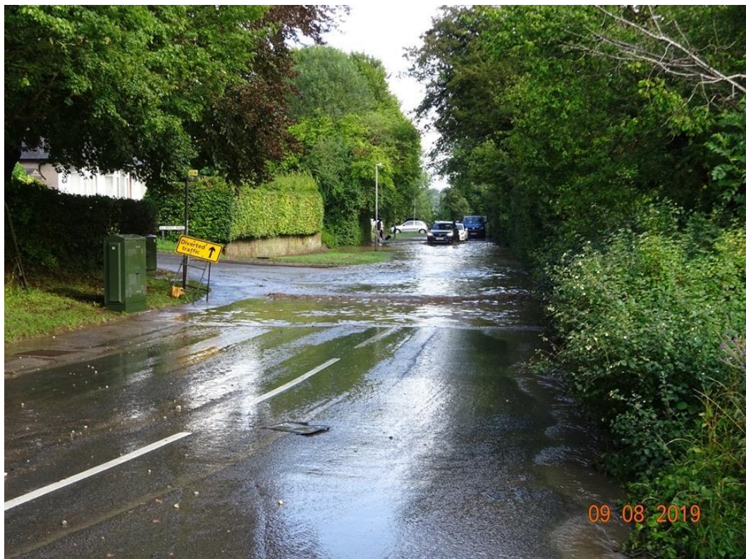
Flooding on Hivings Hill - August 2019
