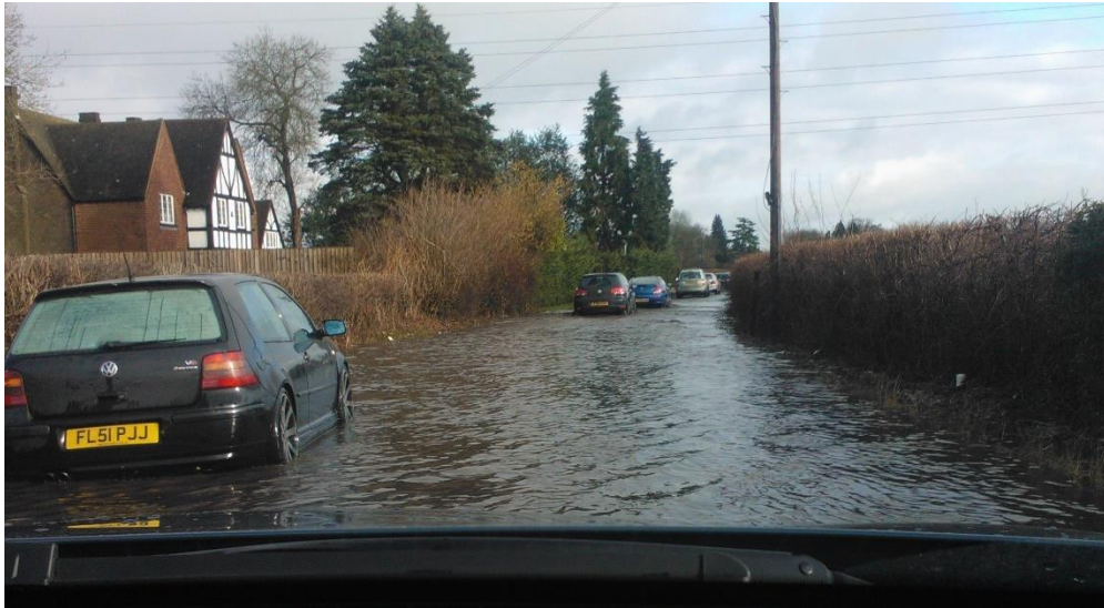
Flooding along Lye Green Road - 2014
