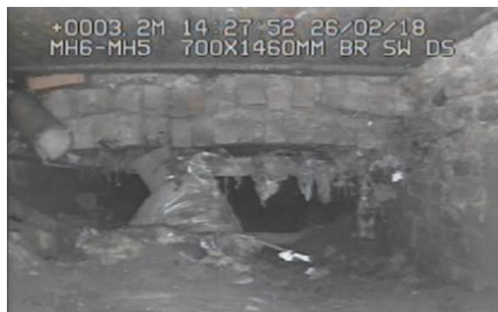
CCTV image of the Vale Brook Culvert
